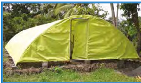
Net Shed Constructed at Barguna Horiculture Centre under ASSSRBP with the supervision of Design & Supervision Consultant
