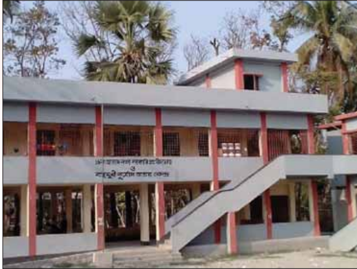
Existing Multipurpose Disaster Shelter (Borhanuddin, Bhola)
