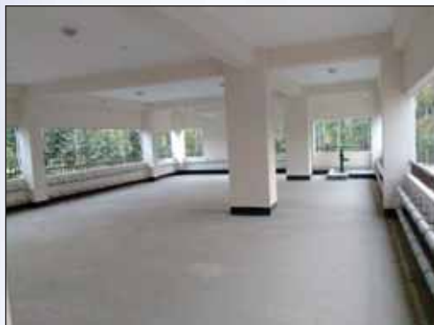
Multipurpose Disaster Shelter (Bhola Sadar)
