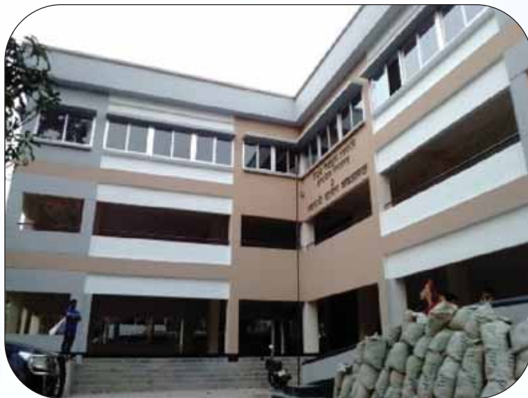
New Multipurpose Disaster Shelter (Bhola Sadar)
