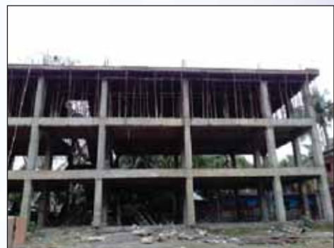
New Multipurpose Disaster Shelter (Lakshmipur)
