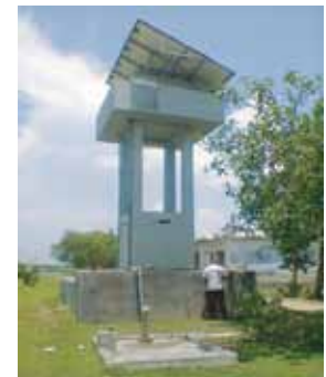
△ Saline Water Purifier at Mithakhali Union, Mongla Upazila in Bagerhat district
