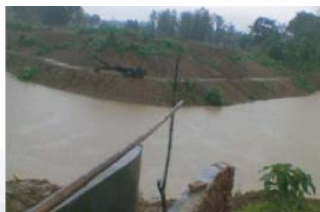
Water reservoir excavation in Ali Kadam Upazila of Banderban district.
