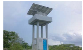
Water dispensing platform run by solar power in Dacope Upazila of Khulna district.
