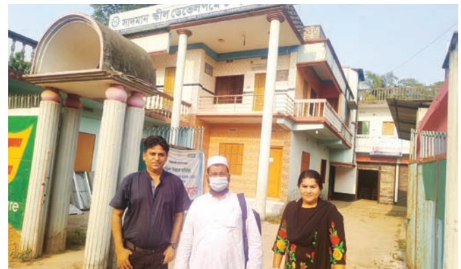
Sadman Skills Development Institute (SSDI), Jessore – a valued client of the MIDAS Technology Transfer Project.
